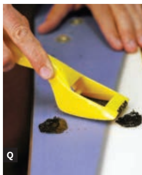
Fig. P: Plug the T-nut holes in the base with hot Metal Grip P-tex repair string. Fig. Q: File down the plugs with the Surform until roughly level. Fig. R: Smooth the plugs perfectly flush with a scraper.
