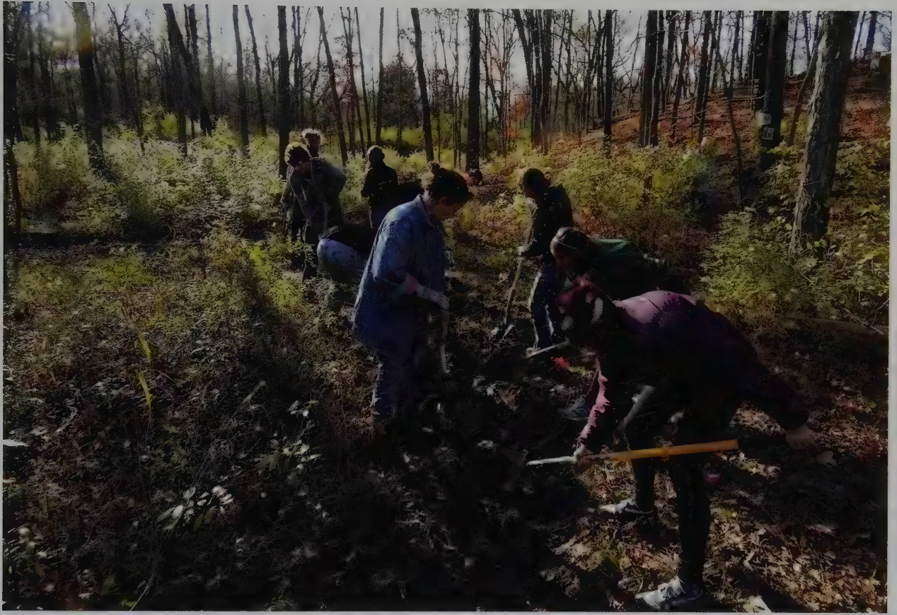
Figure 10.12. At the MacDaniels Nut Grove swales were dug by students to mitigate the effects of seasonal runoff from the uphill Cornell Orchards. Each swale overflows into the next one and eventually flows through a hugelkultur mound and into a vernal pool for eventual evaporation. In this way water is not only managed to avoid causing problems, but the system provides a multitude of wildlife habitat as well.
